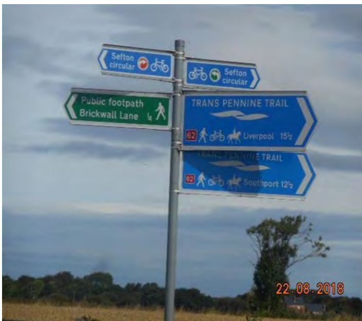
Image 47 Rights of way post with multi directional signs installed on 4m post.
