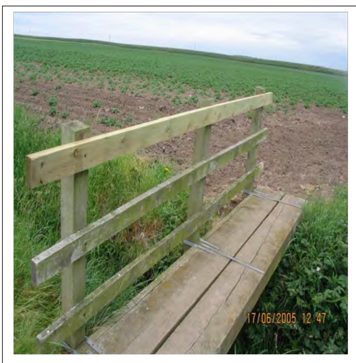
Image 17 repair to handrail undertaken repairs undertaken like for like.
