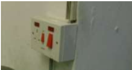
Cooker switch installed
