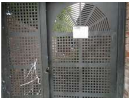
Entrance to Alley /Access to Annex
