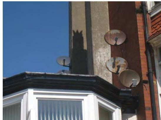
**Deteriorating and numerous poorly located satellite dishes**
