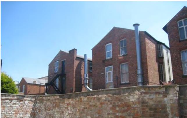
**Significantly sized ductwork gives a poor appearance to rear elevations**
