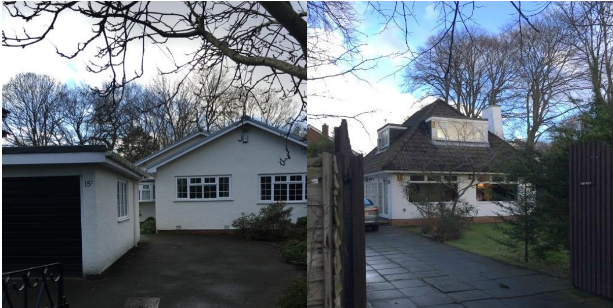
15c Green Lane, a bungalow of no architectural or historic interest
