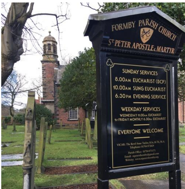
Green Lane entrance to St. Peter's Church showing the original elements including the tower and octagonal bell stage
