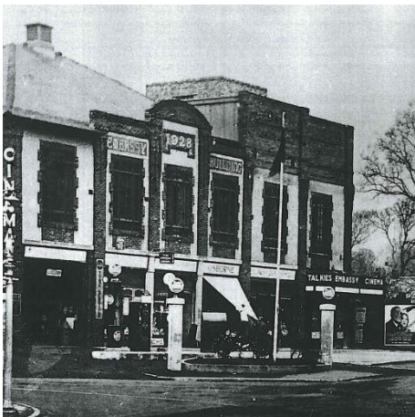
Historic photograph of the Embassy Building, showing an abundance of features and detailing which have since been removed or lost
