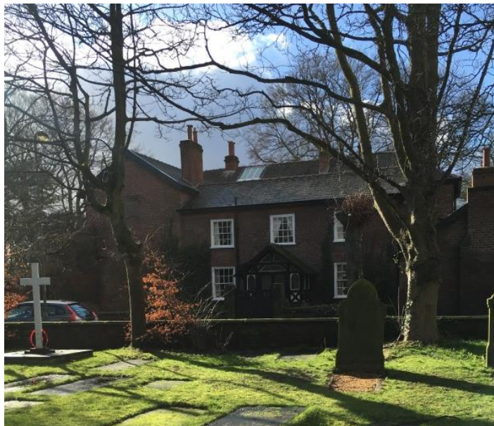
Church House viewed from the church yard of St. Peter's
