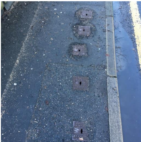
Several service covers located on the pavement at Green Lane could perhaps be incorporated to tidy the public realm
