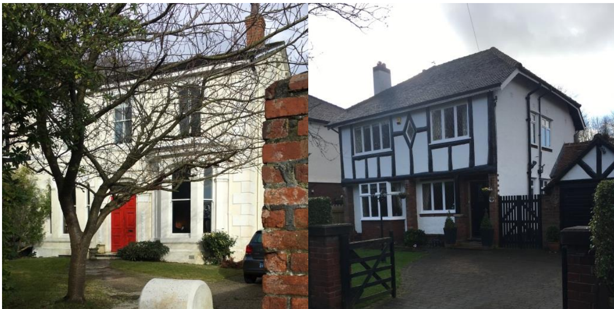
2 and 4 Green Lane are pleasant Victorian homes designed in a Italianate style which is prominent in many of Sefton's urban Conservation Areas
