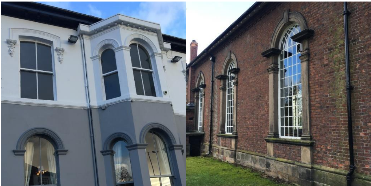
The original sash windows of the Grapes have been well preserved and the curved window surrounds are an attractive edition
