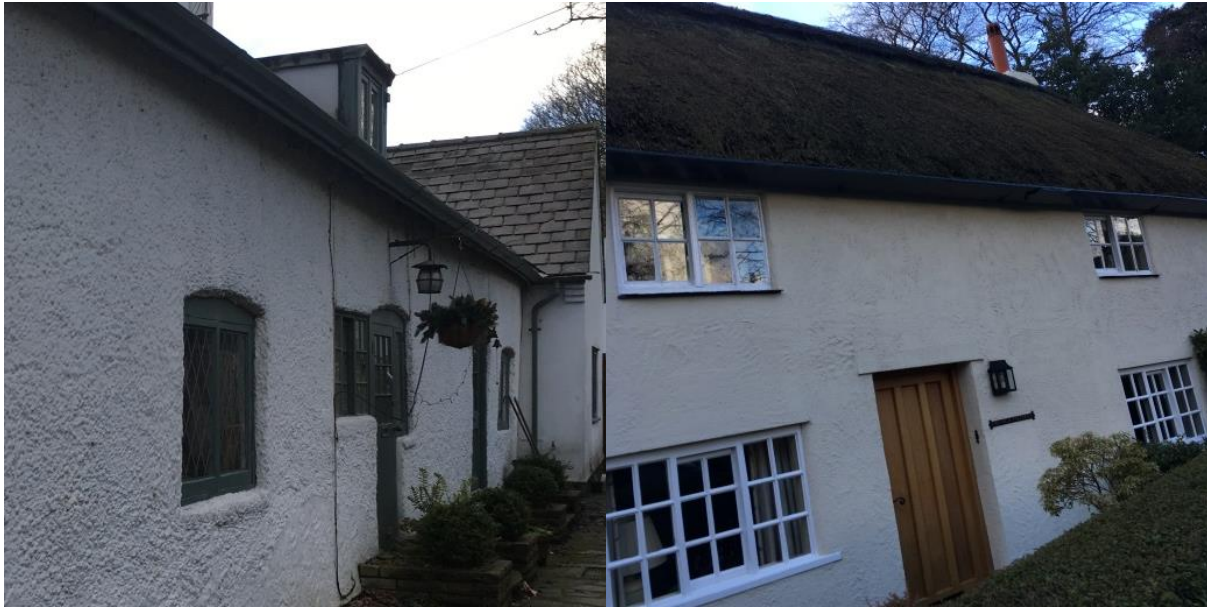
Original casement windows incorporating leadlights with a diamond pattern. Small pane glazing in a similar form is common throughout the Conservation Area
