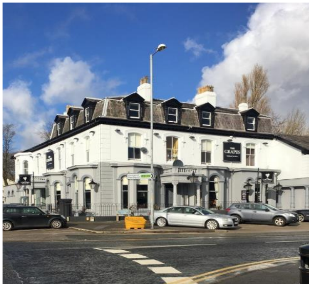
The Grapes Hotel contains elements of French renaissance revival architecture and its prominent location and massing have made it a local landmark
