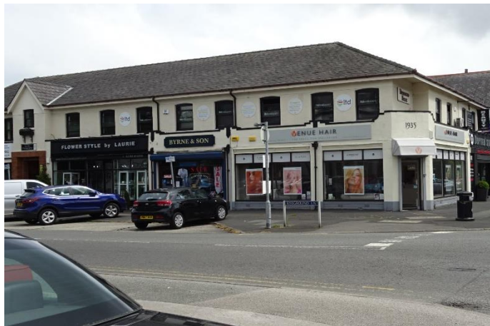
Although Ryeground House has replaced earlier Victorian shops the current style is complimentary of the Embassy Building. Some modern features and proliferation of signage are however unsympathetic to the areas character (photo July 2019)
