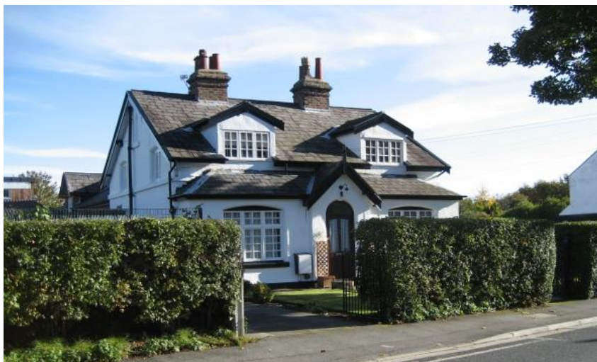
14 Paradise Lane, the original St. Peter's Boys School is an attractive building contrasting between the opposite girls school of the same era
