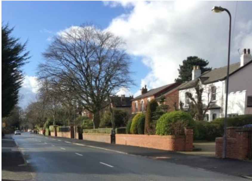
View along Piercefield Road looking east showing Victorian development and significant tree coverage
