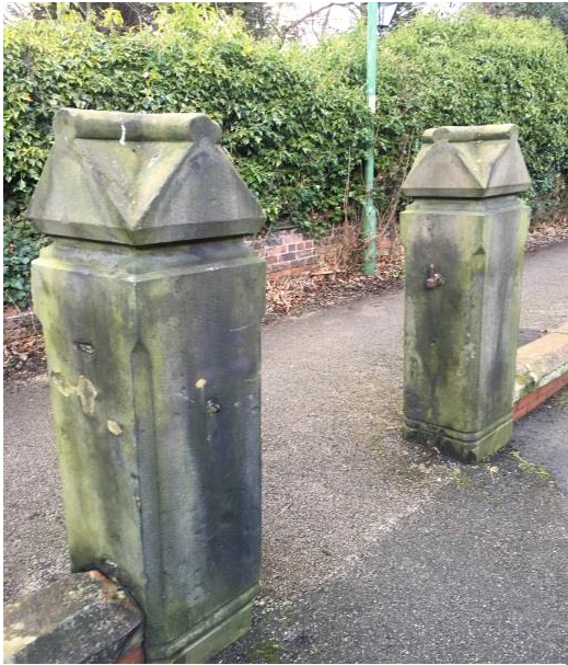
Two sets of gate piers at the boundary of St. Peter's Church at Church Path are in reasonable condition however the gate and adjacent railings have been removed
