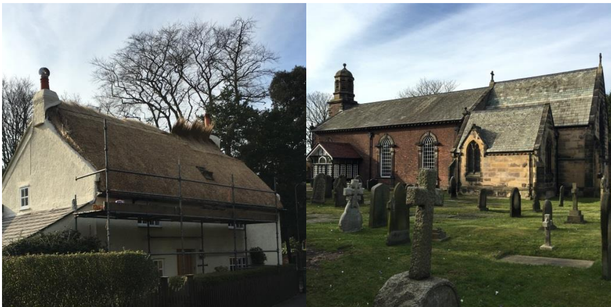
The distinctive thatched roof of 21 Green Lane undergoing maintenance
