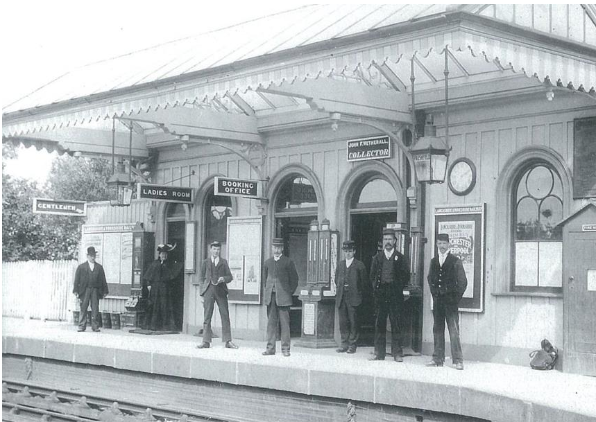
Freshfield Railway Station photographed in 1912, largely unrecognisable against its later 20 th century replacement
