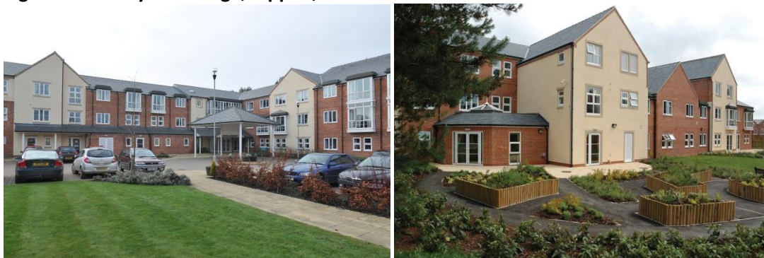
Figure 5.3 Sunnyfield Lodge, Rippon, North Yorkshire
