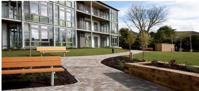
Figure 5.1 Prince Charles House, St Austell, Cornwall
