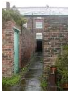
Rear walls along alley from Brunswick Mews
