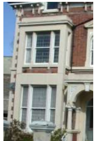
Two-storey square bay
