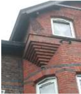
Corbelled brickwork eaves detail on Cambridge Road
