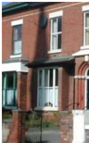
Single-storey square bay
