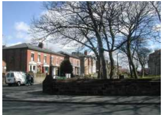
AL1: View of Alexandra Rd across the grounds of Christ Church
