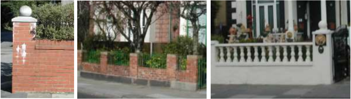
Examples of inappropriate replacement front boundary walls
