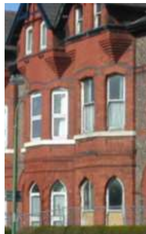
Two-storey canted bays
