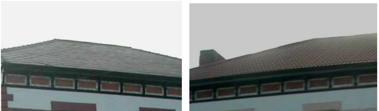
The contrast of texture and colour between a traditional slate roof and a modern tiled roof.
