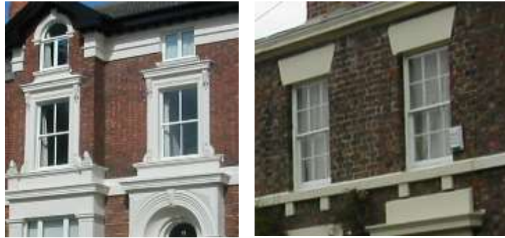
Examples of traditional sliding-sash windows found in the Conservation Area
