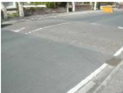
Surface of Waterloo Road
