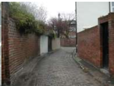
Cobbled surface to the back alley between South View and Olive Road
