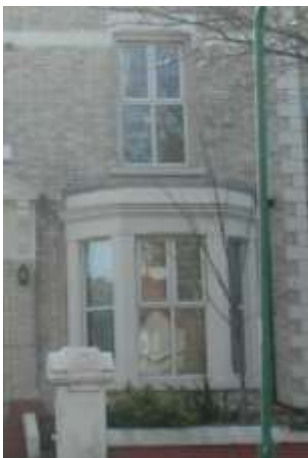
Single-storey canted bay
