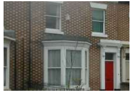
Patterned brickwork for houses on Waterloo Road
