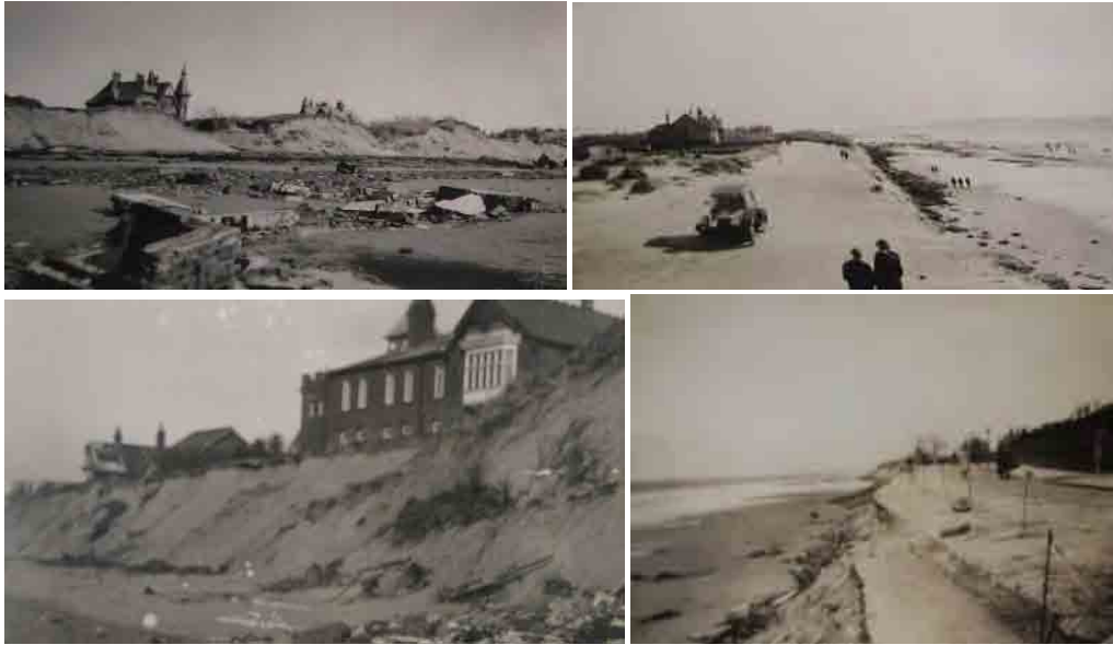
Photographs showing the dramatic coastal erosion and storm damage of the 1920s and 1930s. (Top left) looking towards The Serpentine – The Glen (now demolished) appears on the left; (top right) The Serpentine; (bottom left) Beachside Towers and its neighbour in 1921 before it was swept into the sea; (bottom right) The Serpentine
