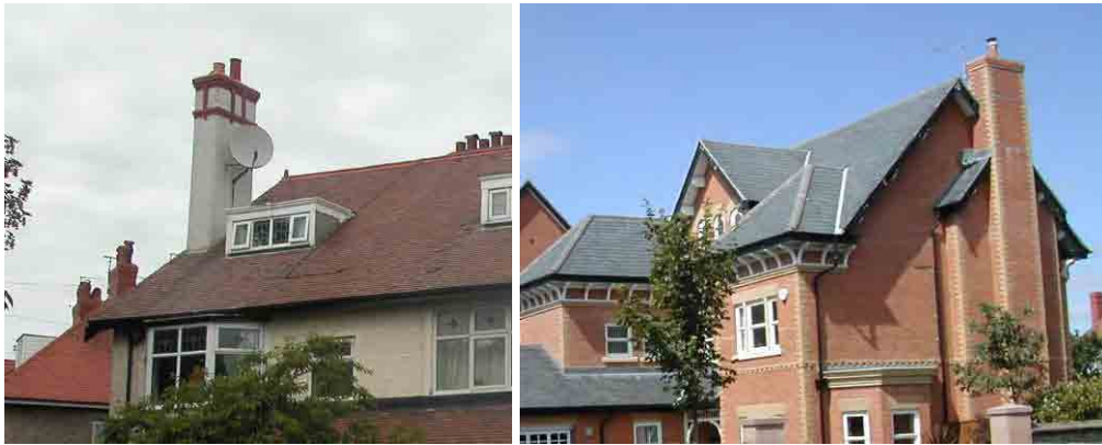
(Left) a large opaque satellite dish positioned obtrusively on a high feature chimney – it is therefore silhouetted against the sky; (right) a smaller grey dish on a new building, tucked away and camouflaged against the leadwork
