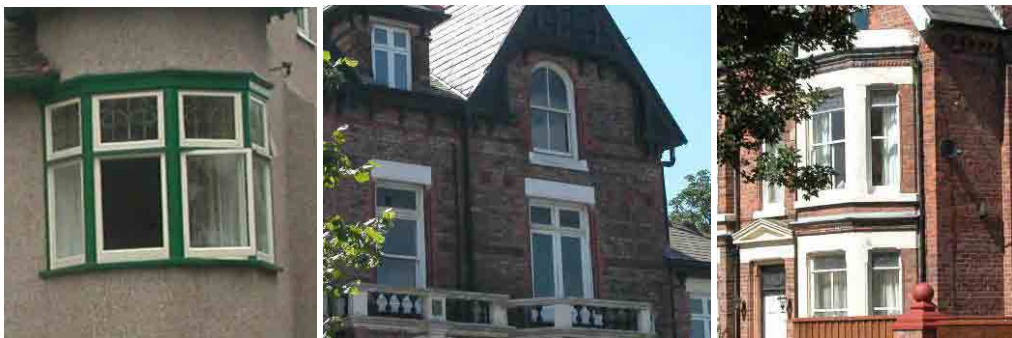
Examples of leaded lights. The middle and the right photographs show instances where leaded lights have been used as part of a sash window.
