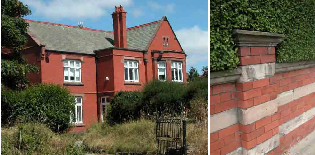
Sandstone used for dressings and in boundary walls.
