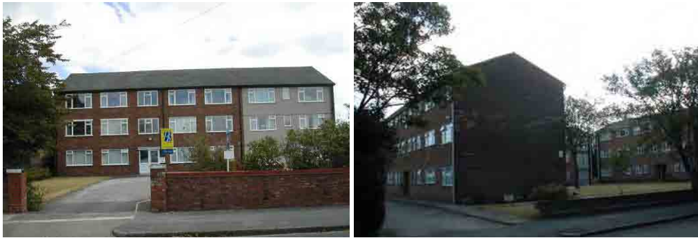
Flats built around the 1970s
