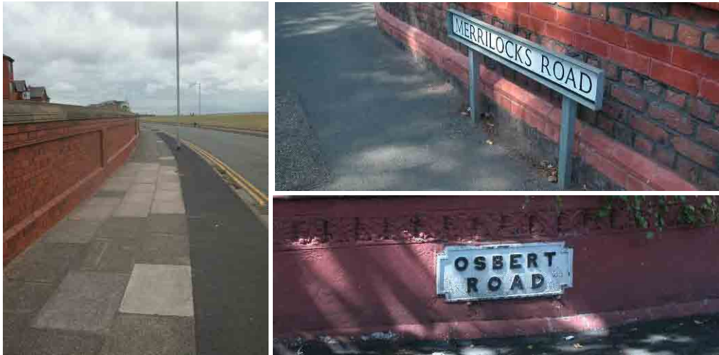
(Left) poor quality paving; (right) modern and original street name signage
