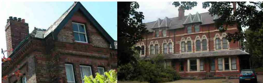
Brickwork detailing: (Left) terracotta detailing to eaves; (right) polychromatic brick banding
