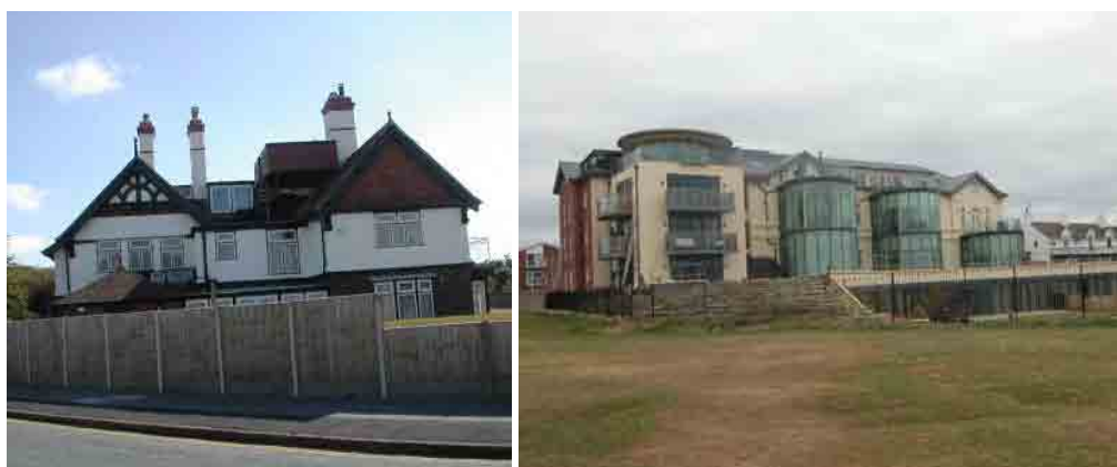
Small and large scale unsympathetic extensions. The left example shows the dramatic effect a relatively small addition to a roof can have. The right hand photograph shows a dramatic extension / alteration to a historic building that entirely obliterates its original character from the sea facing side.
