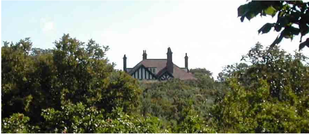
View across Key Park showing the contribution which chimneys make to the character of the area
