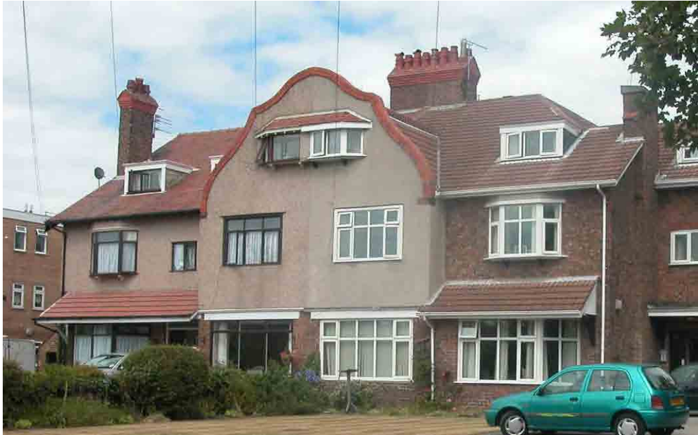
The dramatic effect changing roofing materials can have on the visual balance of a semi-detached or terraced group.
