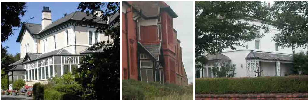
Porches, conservatories and canopies within the conservation area
