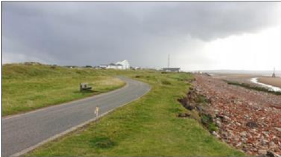
Figure 3: Proximity of coastal path to eroded cliff edge.
