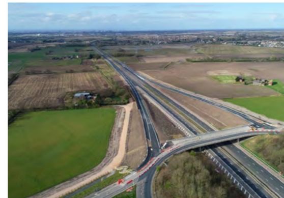
M58 Junction works
