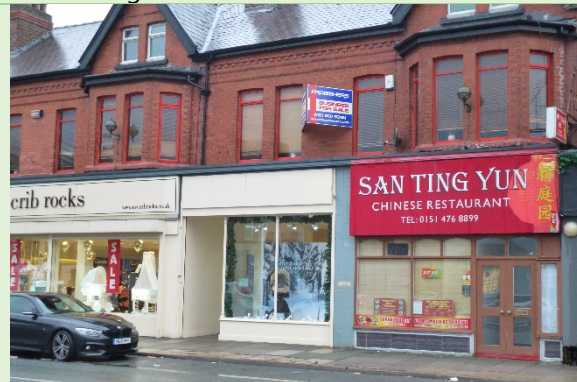
Figure 4: Retail units on Crosby Road North in January 2019
