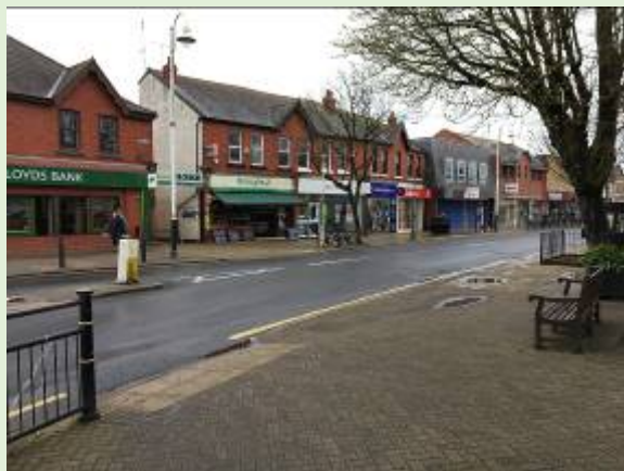
Figure 1: Commercial units on Chapel Lane viewed in March 2020
