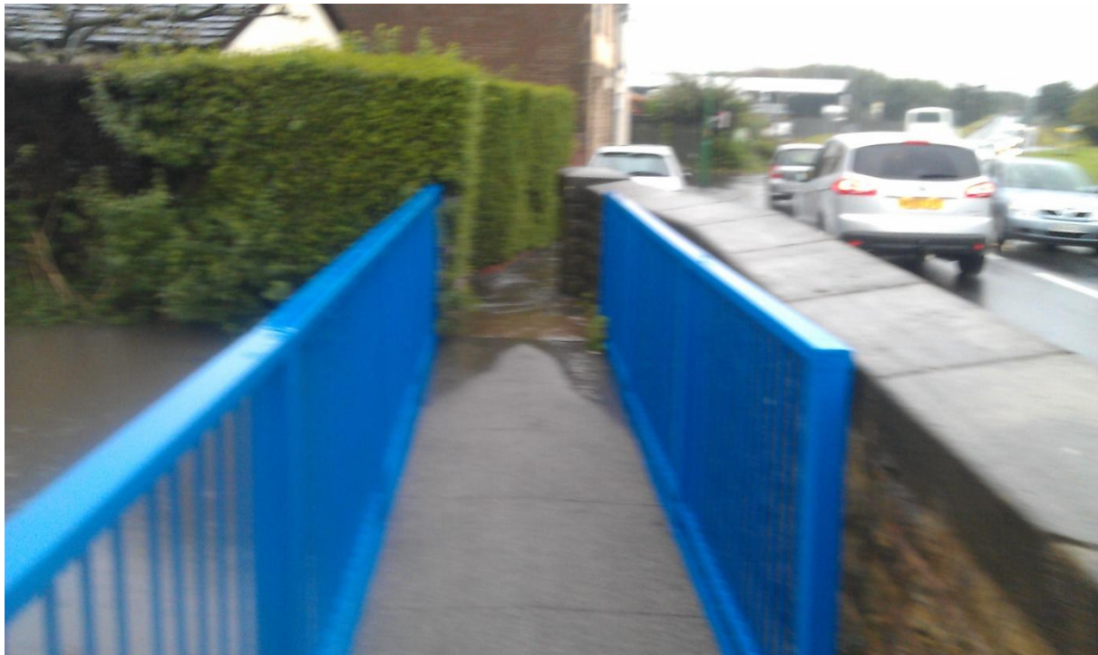
Figure 15: Dover’s Brook flooding into Sefton Lane, taken 24/09/2012
