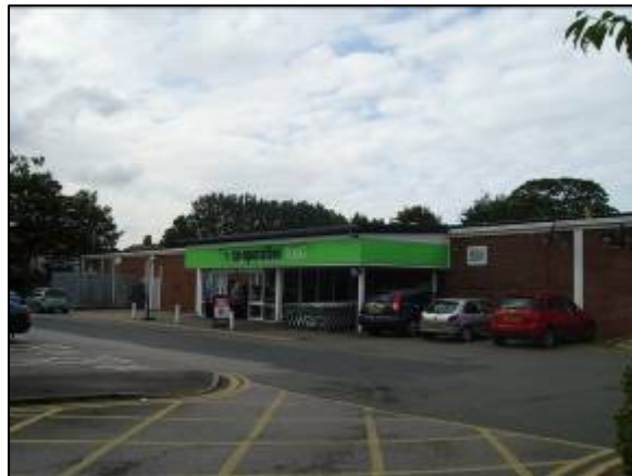
Co-op Foodstore, Station Road
