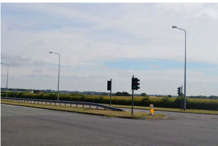
VP7. View looking northeast across the site from A59, southwest corner of site
