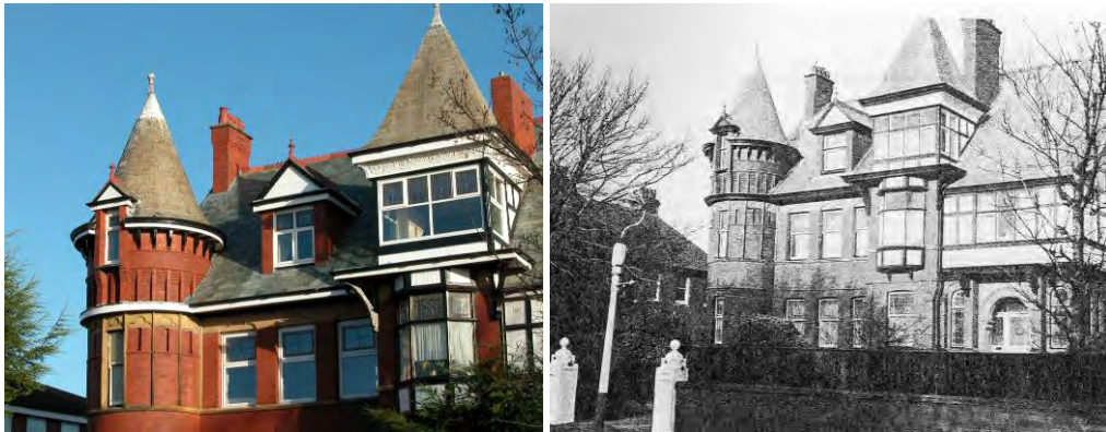
These photographs illustrate the negative impact of changes to windows, timberwork, chimneys and panelling within the past 20 years. In this time the front boundary wall and gateposts have also been removed. The trees and shrubs to the front garden have also been lost.
