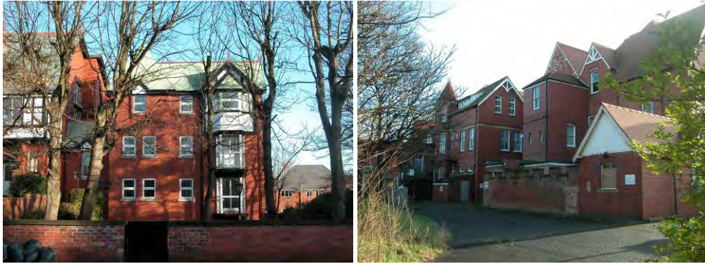
Significant extensions to 3 Grosvenor Road and to the rear of Terra Nova
