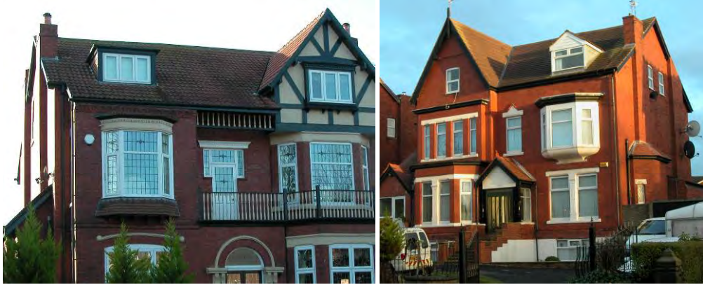
The negative effect that replacement pantile (left) and concrete tile (right) roof coverings have on the appearance of a building.
