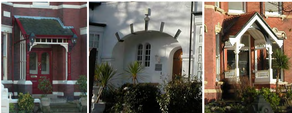
Doors, porches and canopies within the conservation areas
