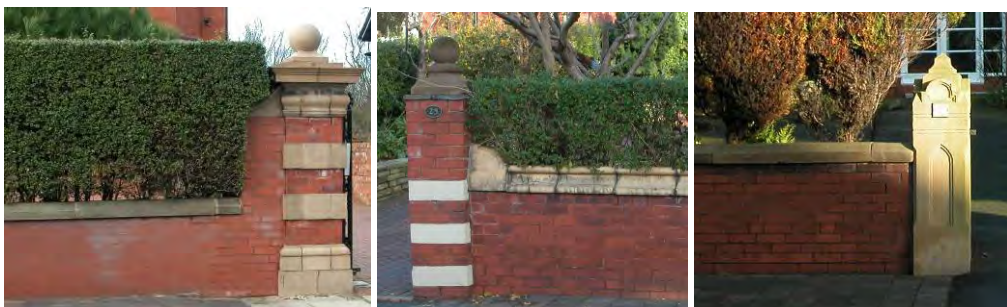
Gate piers within the conservation areas
