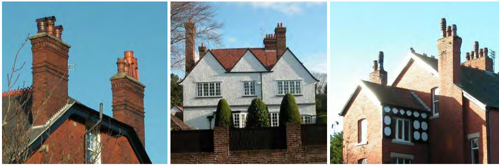
Chimneys within and adjacent to the conservation area
