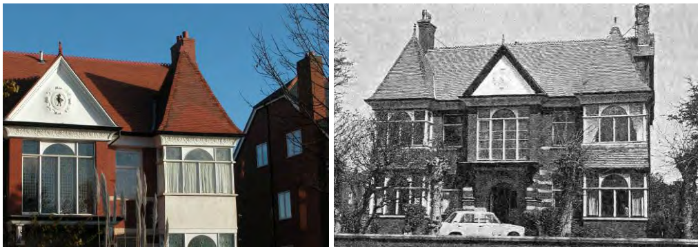
The above photographs illustrate the changes to no. 5 Grosvenor Road. The leaded windows have been double glazed, leaving one smooth plate of glass on the outside. Although the leaded comes have been retained, or replicated on the inside one of the essential characteristics of the glazing, namely the shimmering faceted nature of the windows in the sunlight, has been lost. The hung tiles to the square bays have also been replaced by comparatively crude render and the tops of the chimneys removed.
