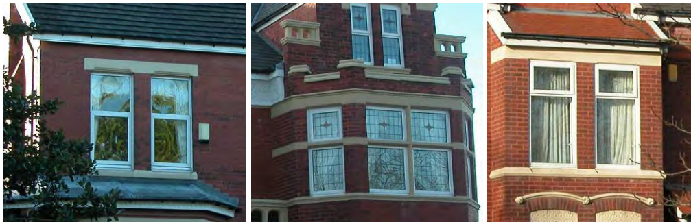
Replaced windows in the conservation area
