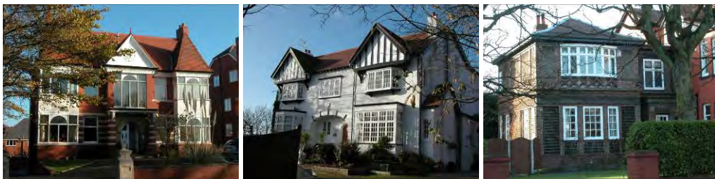
Buildings built using Arts and Crafts or Domestic Revival influences
