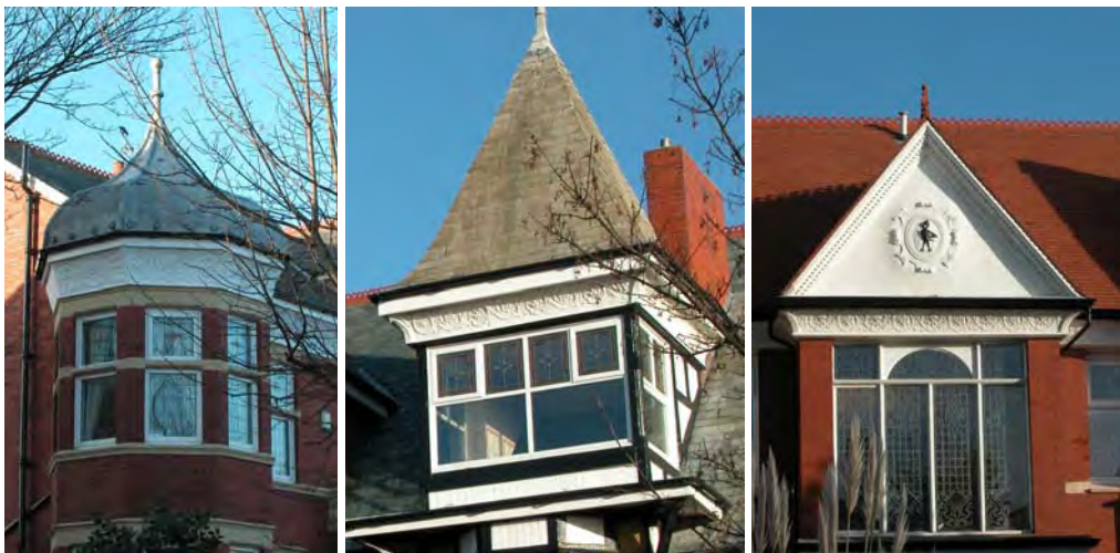
The same decorative plaster frieze is seen on 3 otherwise different buildings on Grosvenor Road, indicating that they were probably by the same developer.
