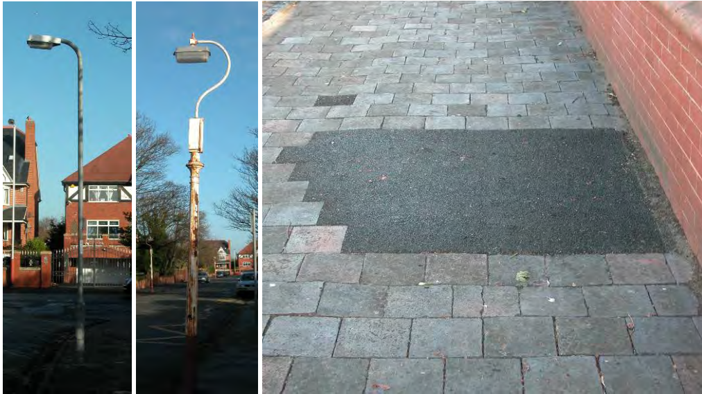
(Left) An example of a poor quality, modern lamppost; (middle) an example of an older cast-iron lampposts, with a modern alteration – the original part of this lamppost could be used as a model for any replicas in the conservation area; (right) a crude repair to the attractive clay pavings.
