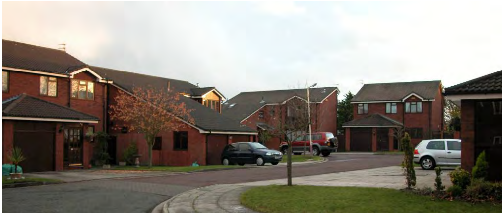
Modern cul-de-sac just outside, but affecting the setting of the conservation area.
