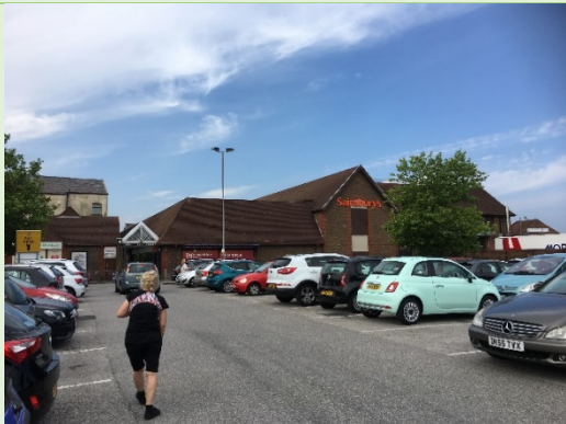
Figure 3: The well-used Allengate car park is located adjacent to Sainsbury's and Moor Lane at June 2018
