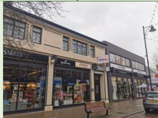
Figure 4: Recently refurbished shop units on Moor Lane at March 2020
